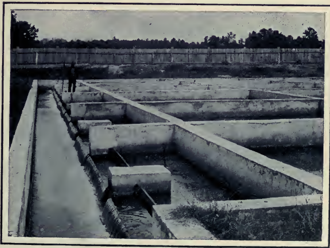
DISCHARGE-WEIRS, SEPTIC TANKS, BIRMINGHAM, ALA. (From Municipal Journal and Engineer .)
